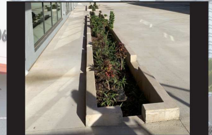
Completed At-Grade Biofilter
