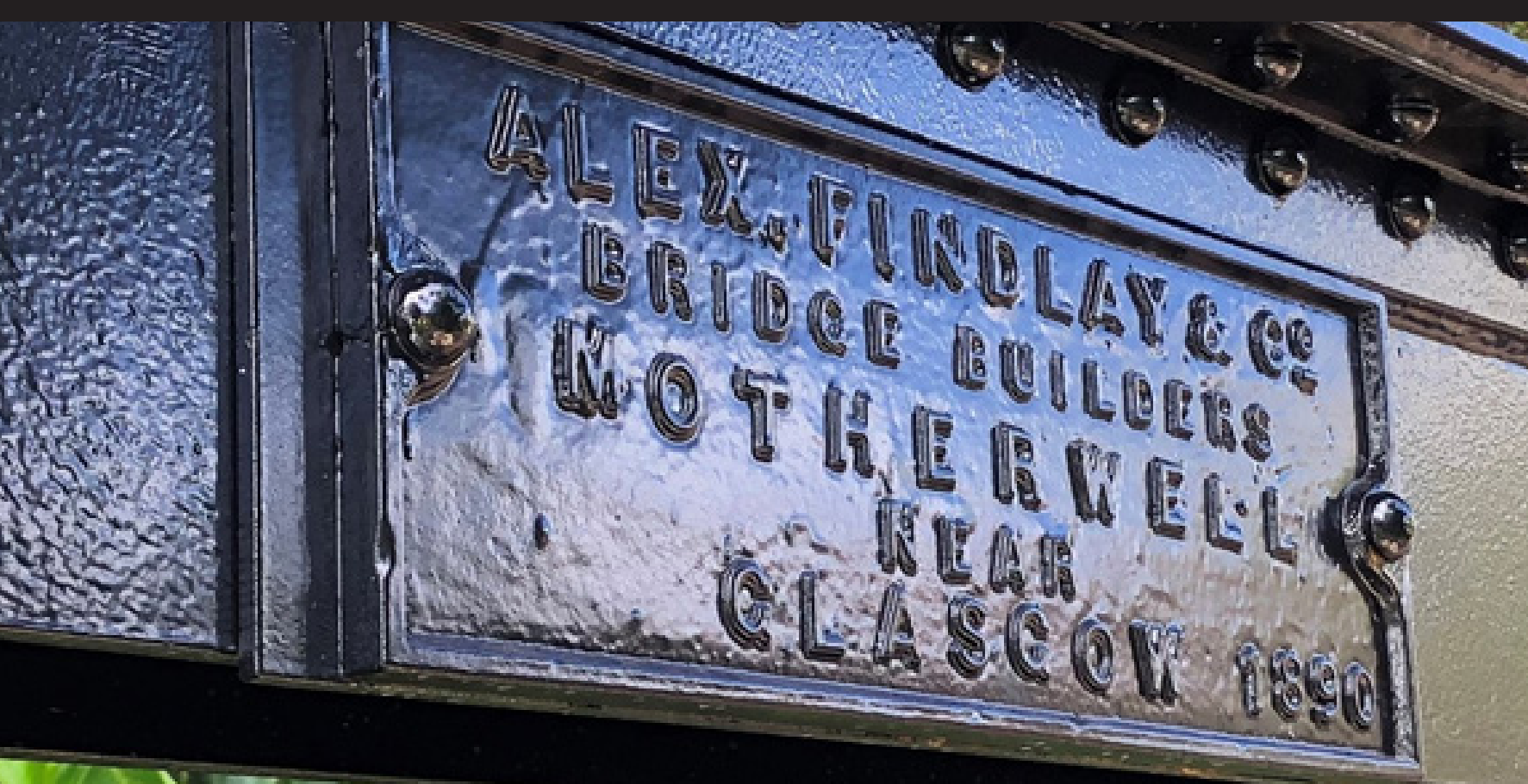
Original plaque that is attached to the top truss chord
